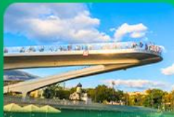
Floating Bridge Moscow
